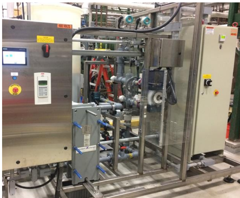
Figure 1: Zimpro® electro-oxidation (ZEO) pilot unit.
